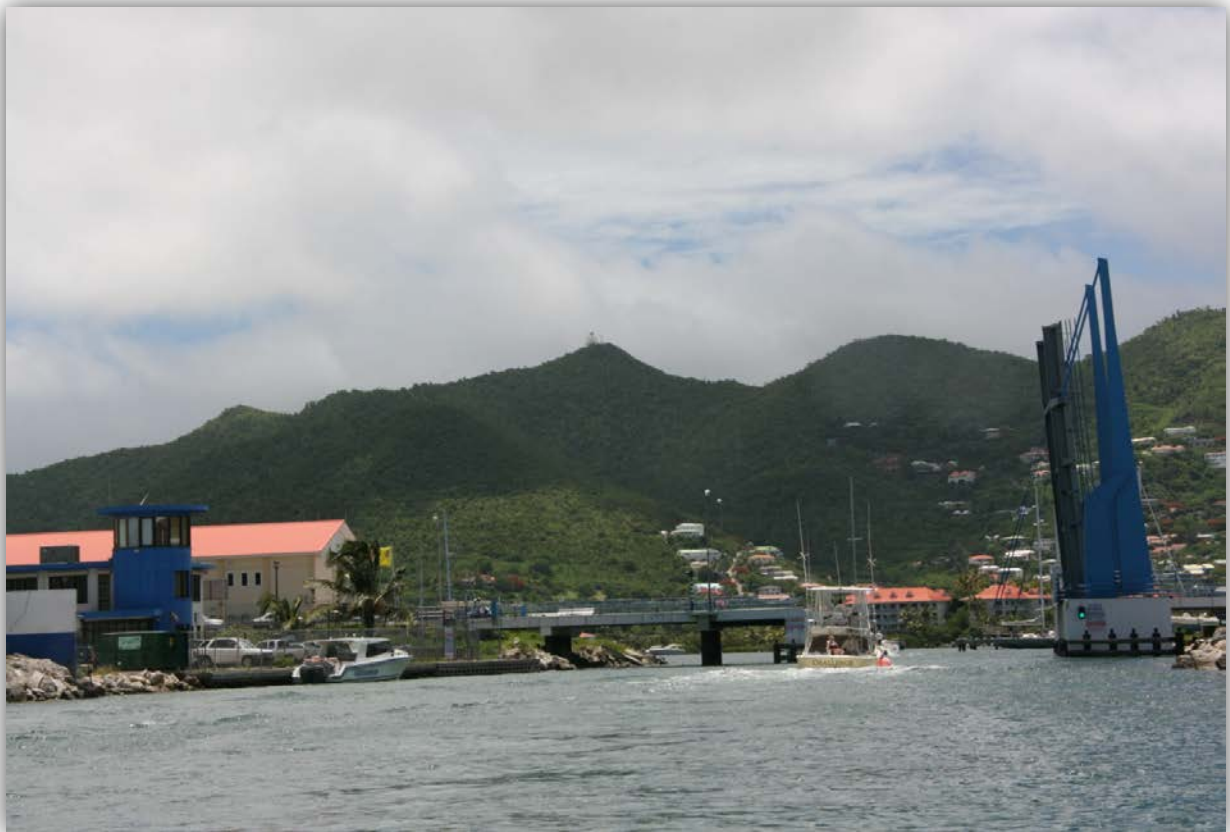
SIMPSON BAY BRIDGE~DUTCH SIDE SEAWALL DOCK FOR CUSTOMS AND IMMIGRATION (L)
