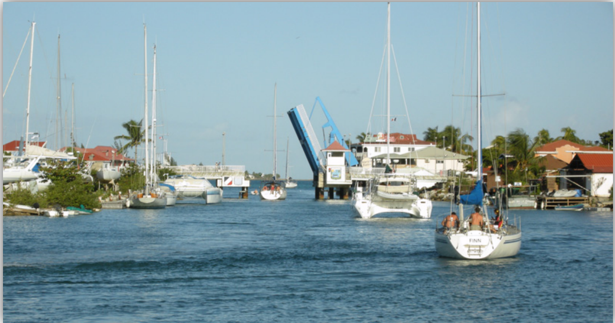
SANDY GROUND BRIDGE~FRENCH SIDE: THE OPENING IS 32' WIDE BUT THE DEPTH IS LIMITED
