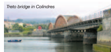
Treto bridge in Colindres
